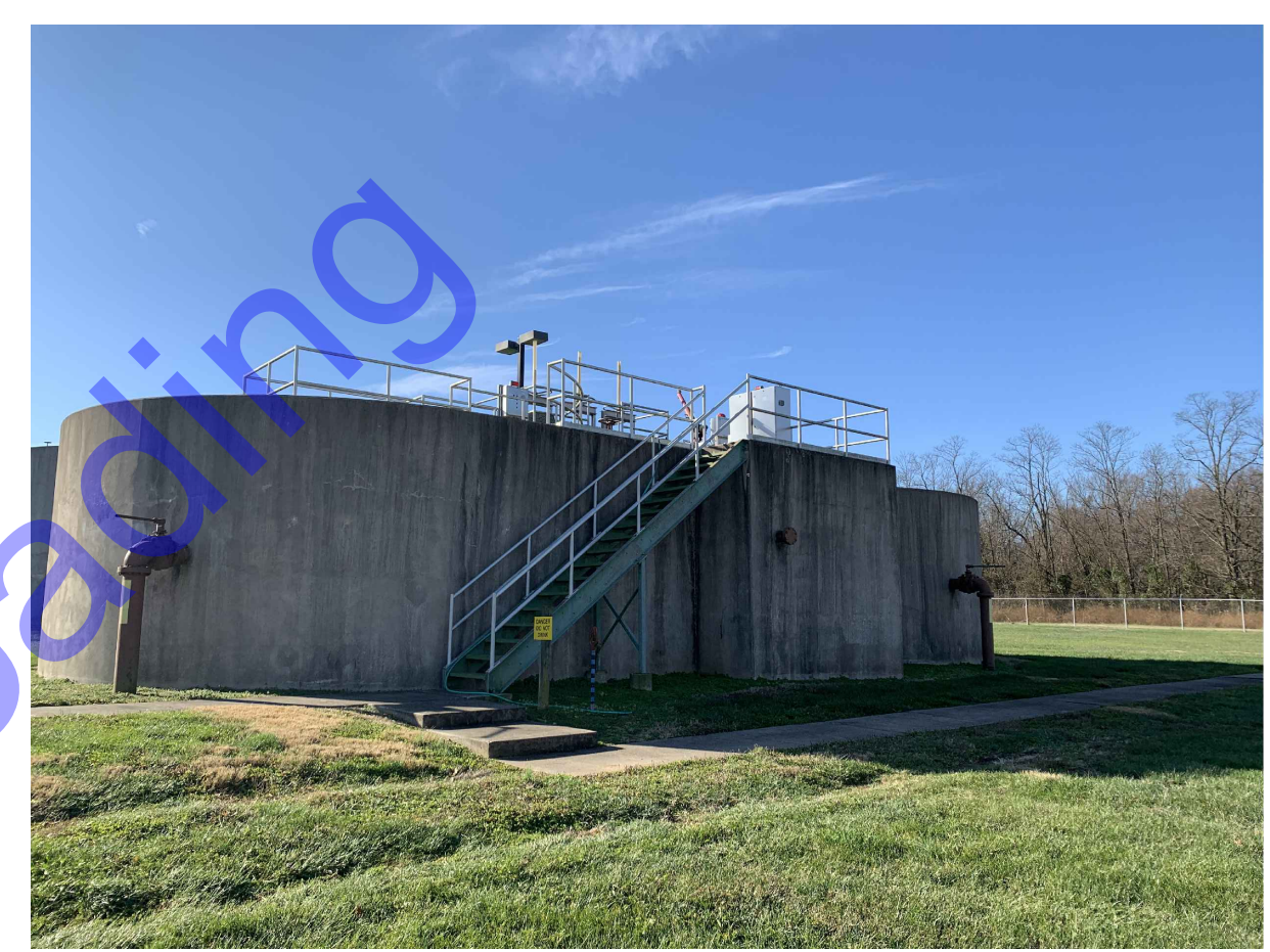
STRUCTURE NORTH VIEW
