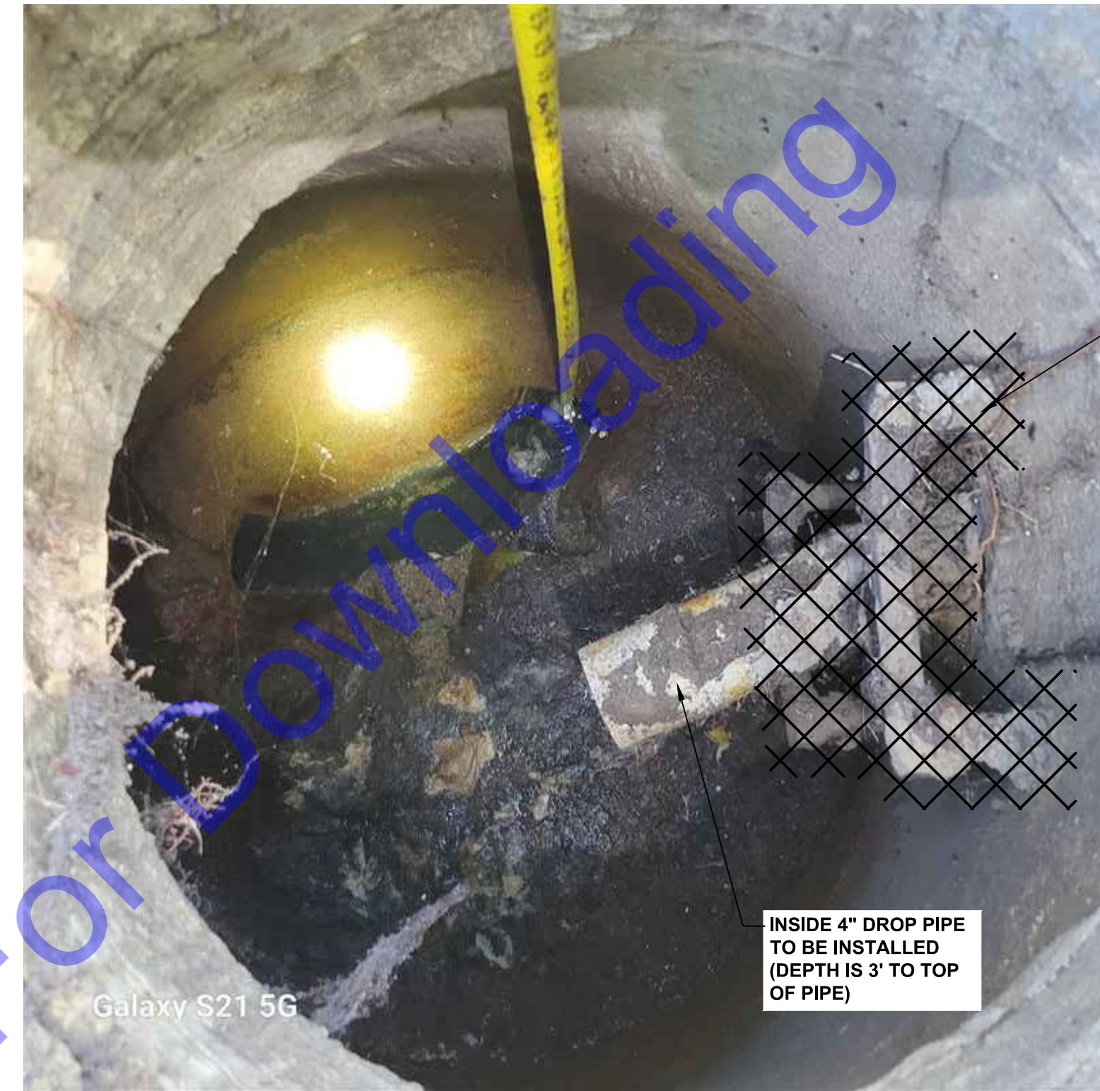
EXISTING MH-15 (SEE DRAWING C1 FOR LOCATION)
