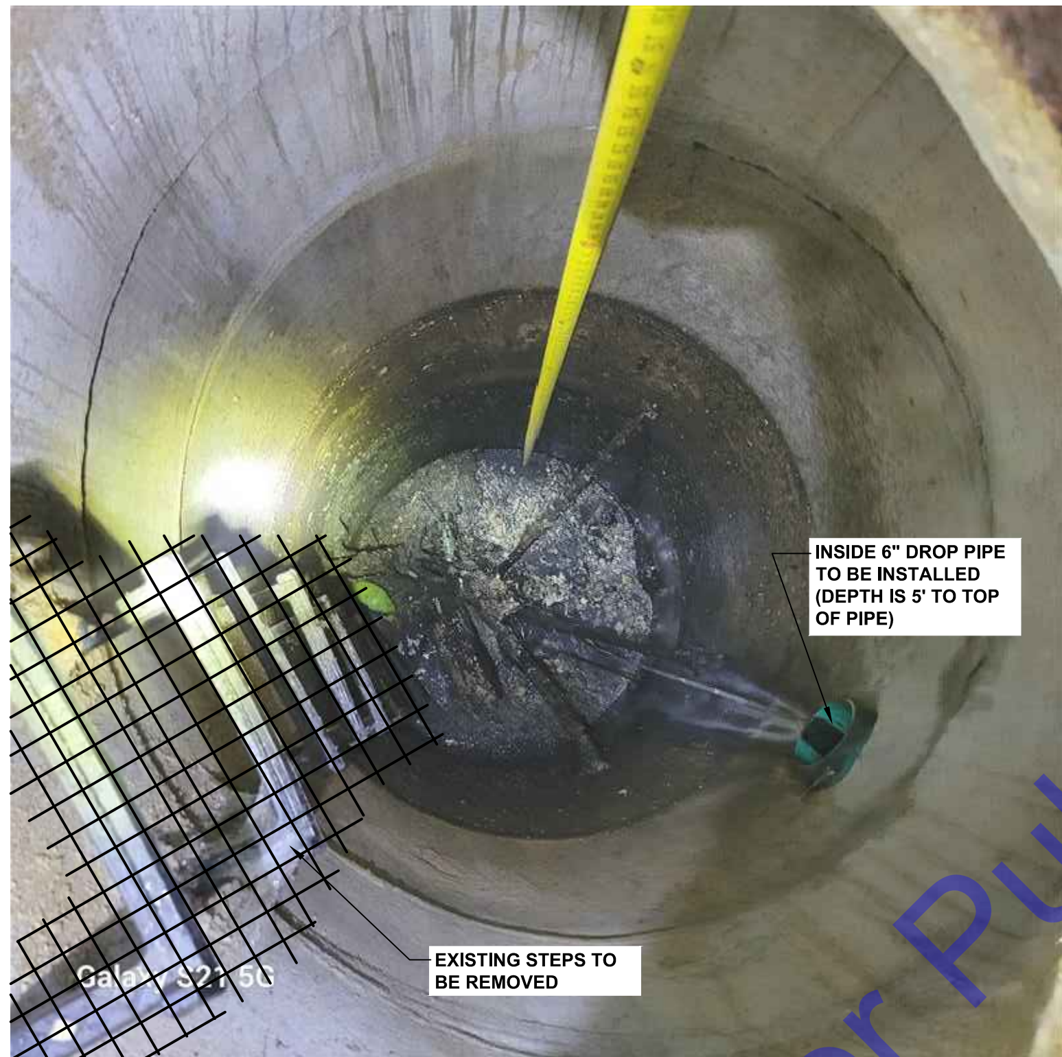
EXISTING MH-21 (SEE DRAWING C2 FOR LOCATION)
