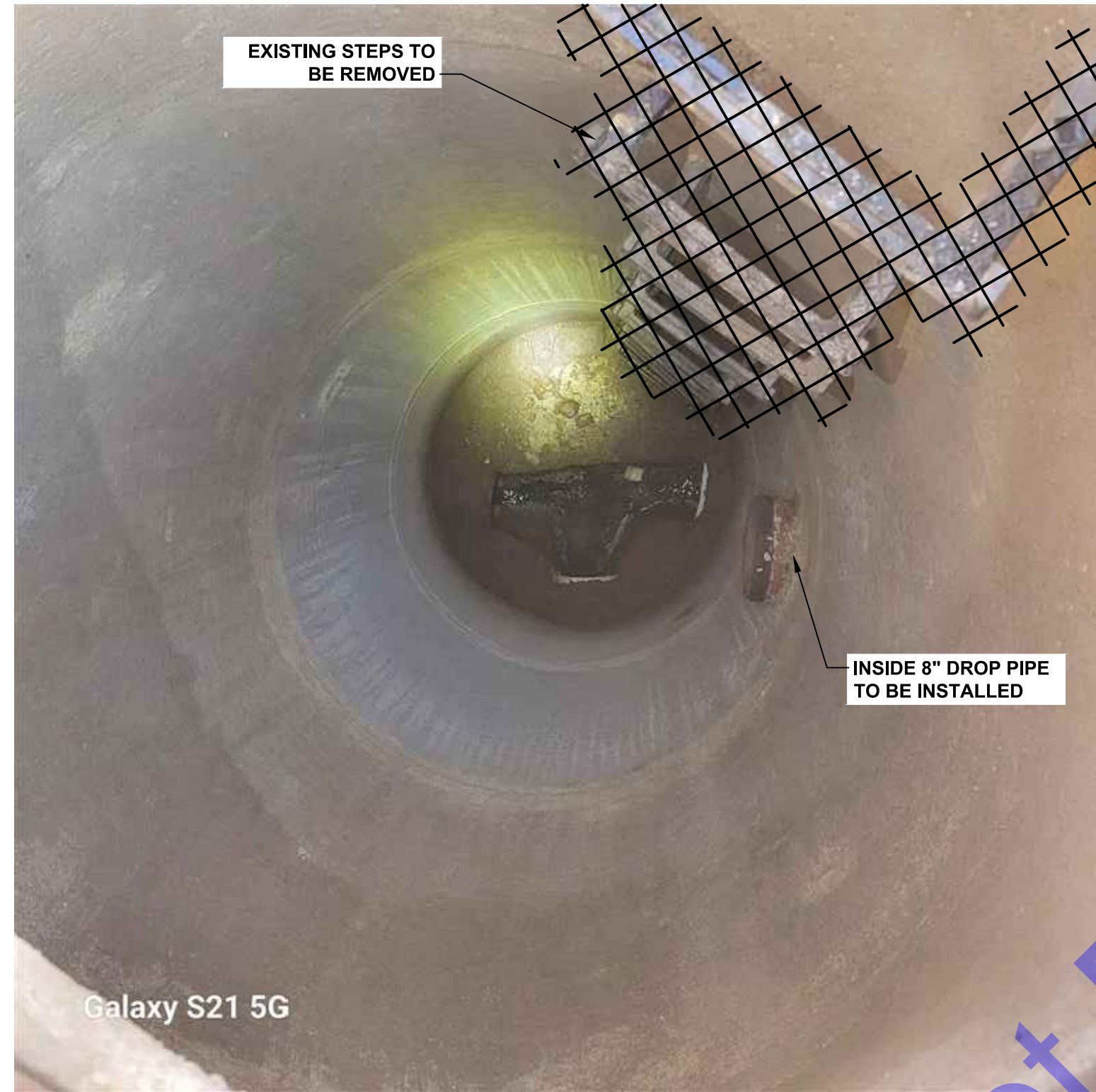
EXISTING MH-14 (SEE DRAWING C1 FOR LOCATION)
