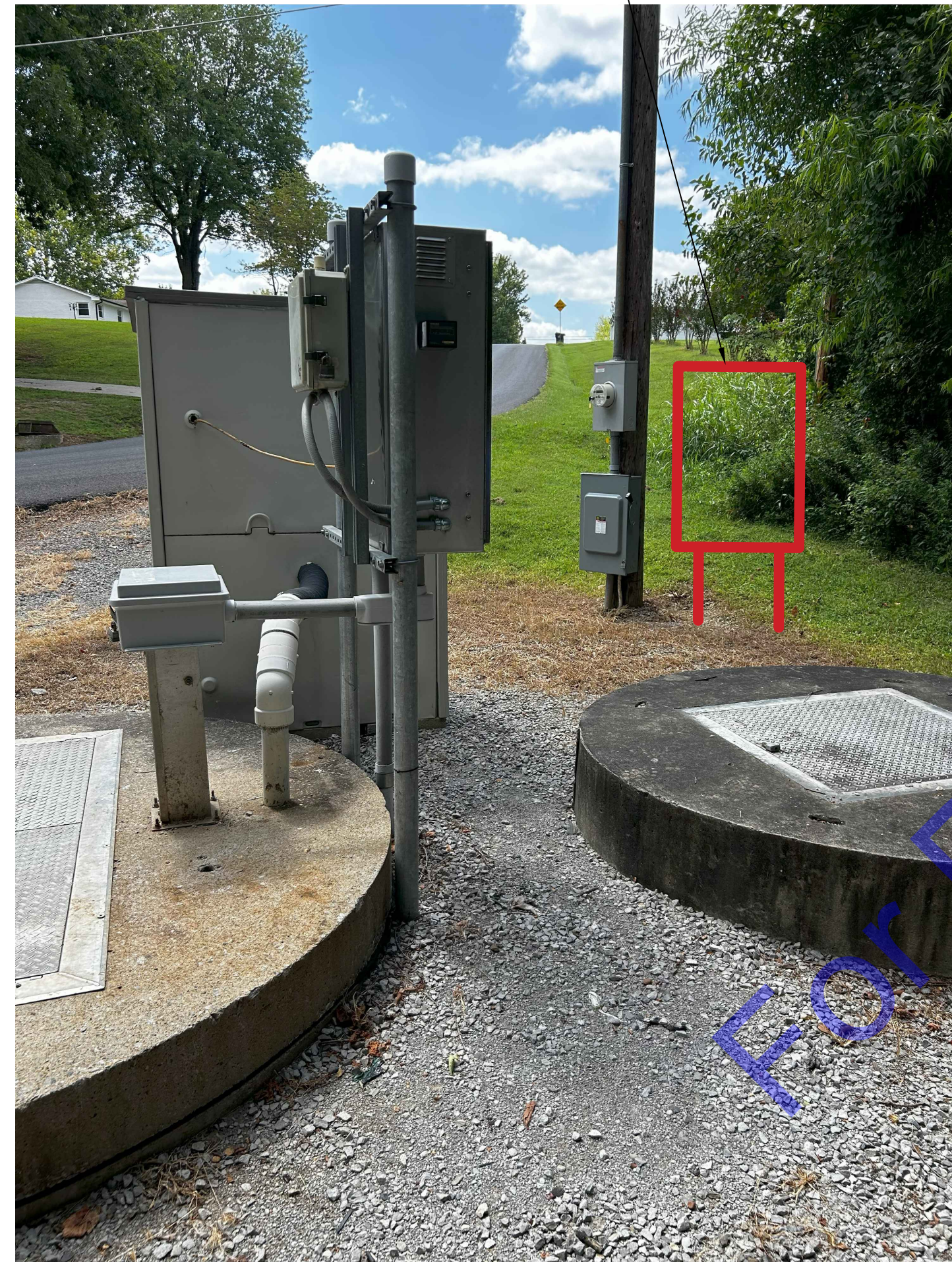
PROPOSED LOCATION OF NEW 200A AUTOMATIC TRANSFER SWITCH
