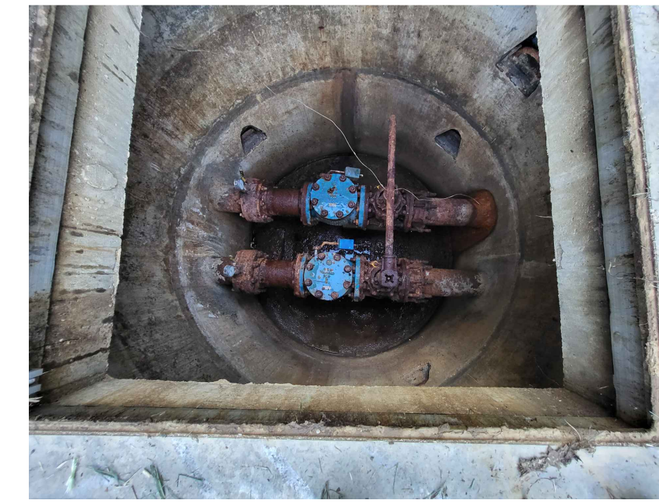
LIFT STATION #2 VALVE VAULT INTERIOR VIEW
