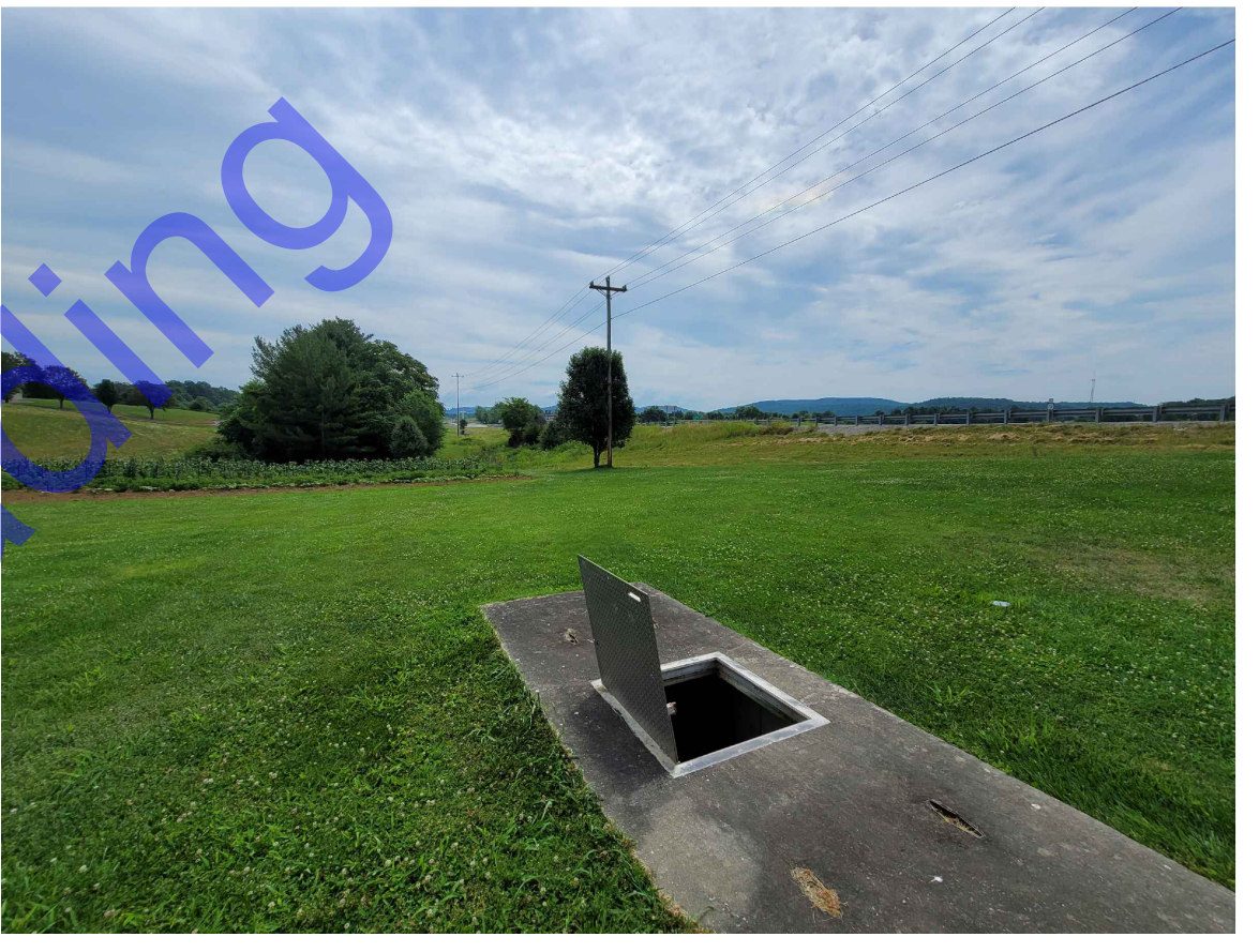
METER 6: EX. METER (TO BE REPLACED) FACING EAST PHOTO 6 NOT TO SCALE
