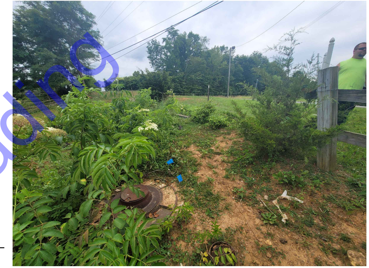
METER 21: EX. METER (TO BE INSTALLED ON 12" MAIN) FACING SOUTH
