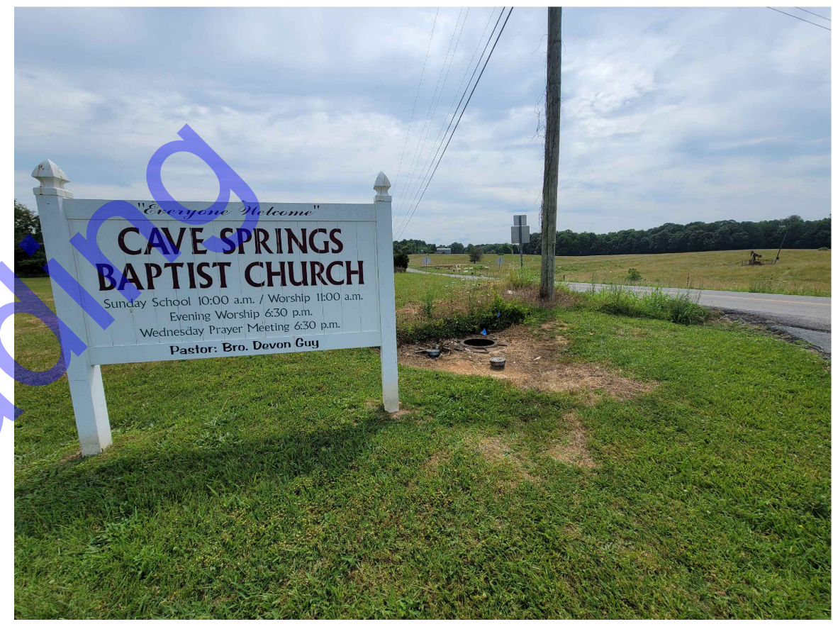
METER 3: EX. METER (TO BE REPLACED) FACING EAST PHOTO 3 NOT TO SCALE
