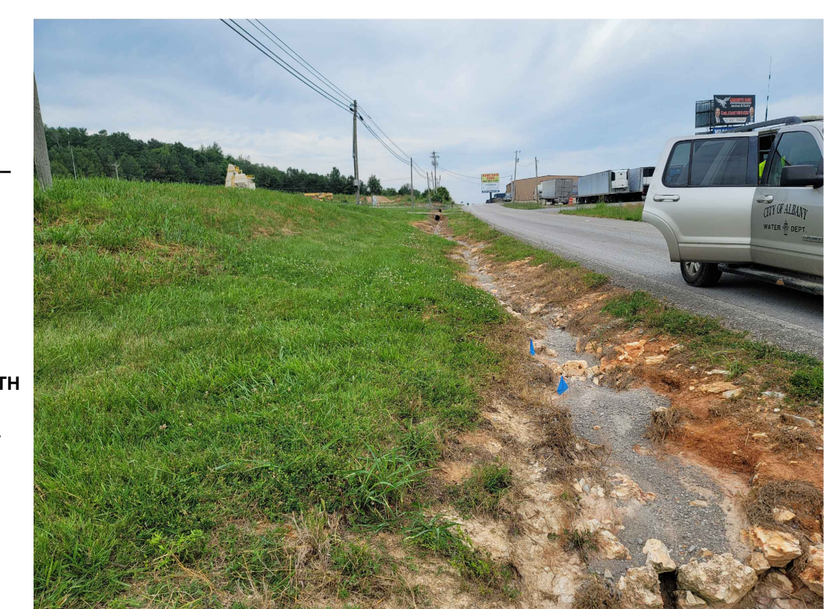
METER 35: NEW METER FACING SOUTH PHOTO NOT TO SCALE 35
