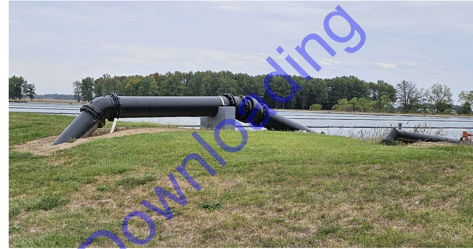
EXISTING FORCE MAIN EFFLUENT DETAIL - REFERENCE PICTURE
