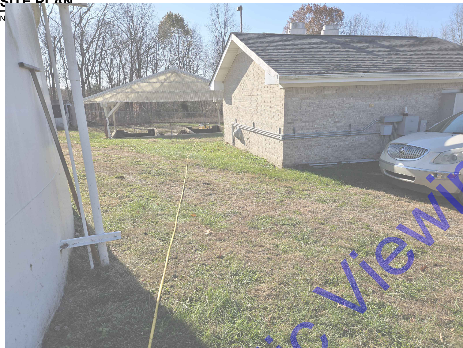
VIEW OF LAB/OFFICE FROM AERATION SYSTEM
