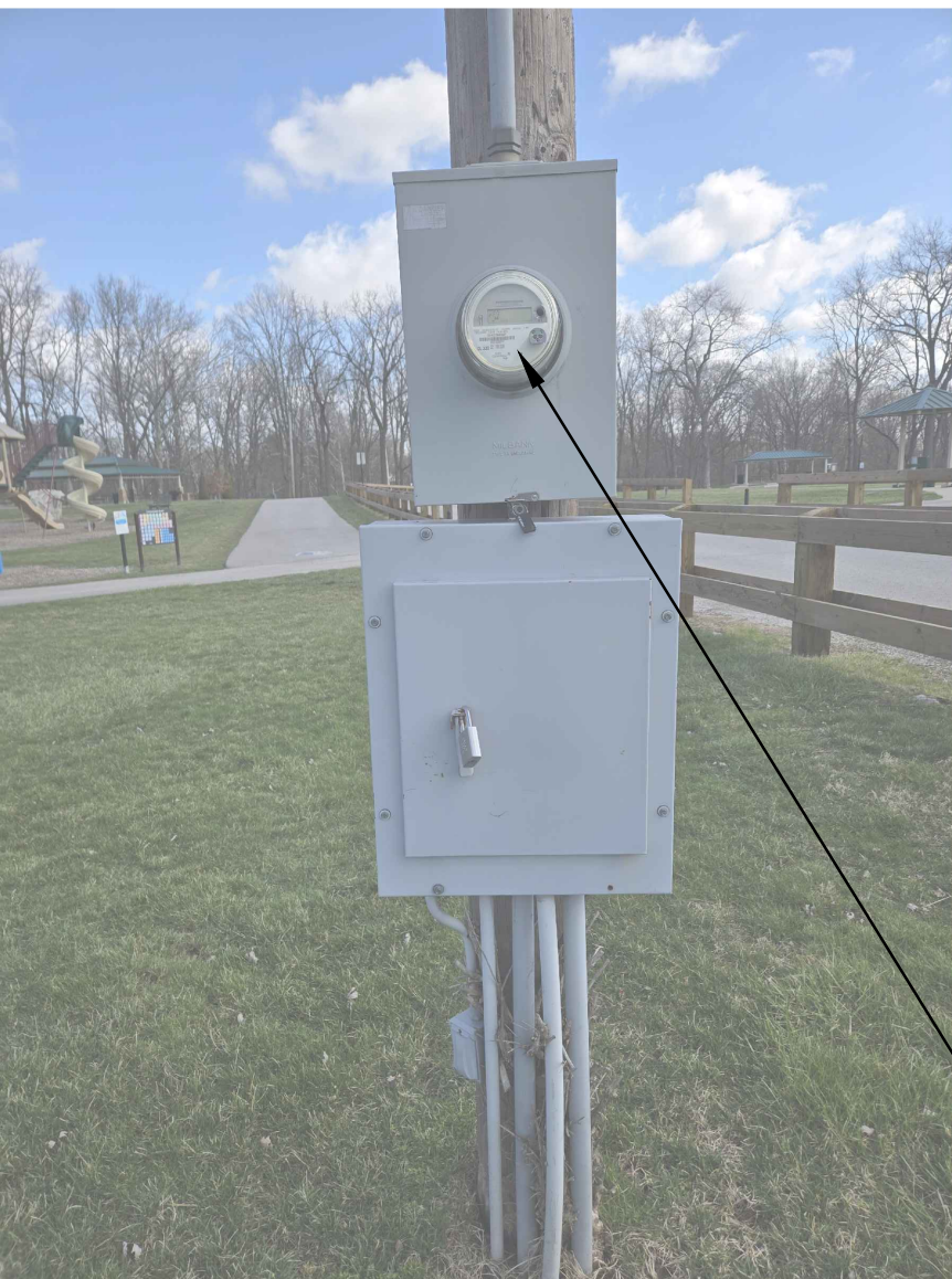
LIFT STATION METER BASE AT ARBUCKLE ACRES PARK
